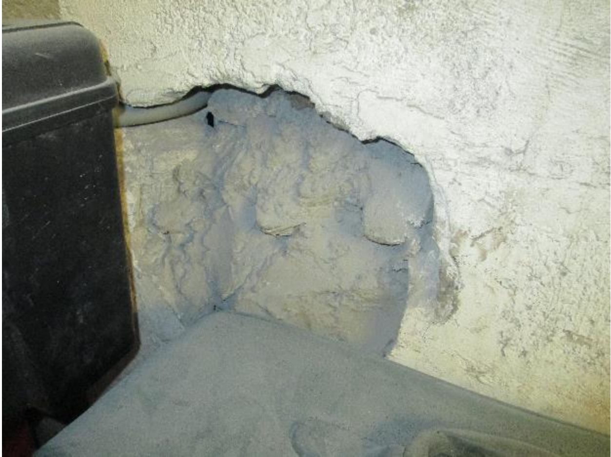
Repairs interior walls.
