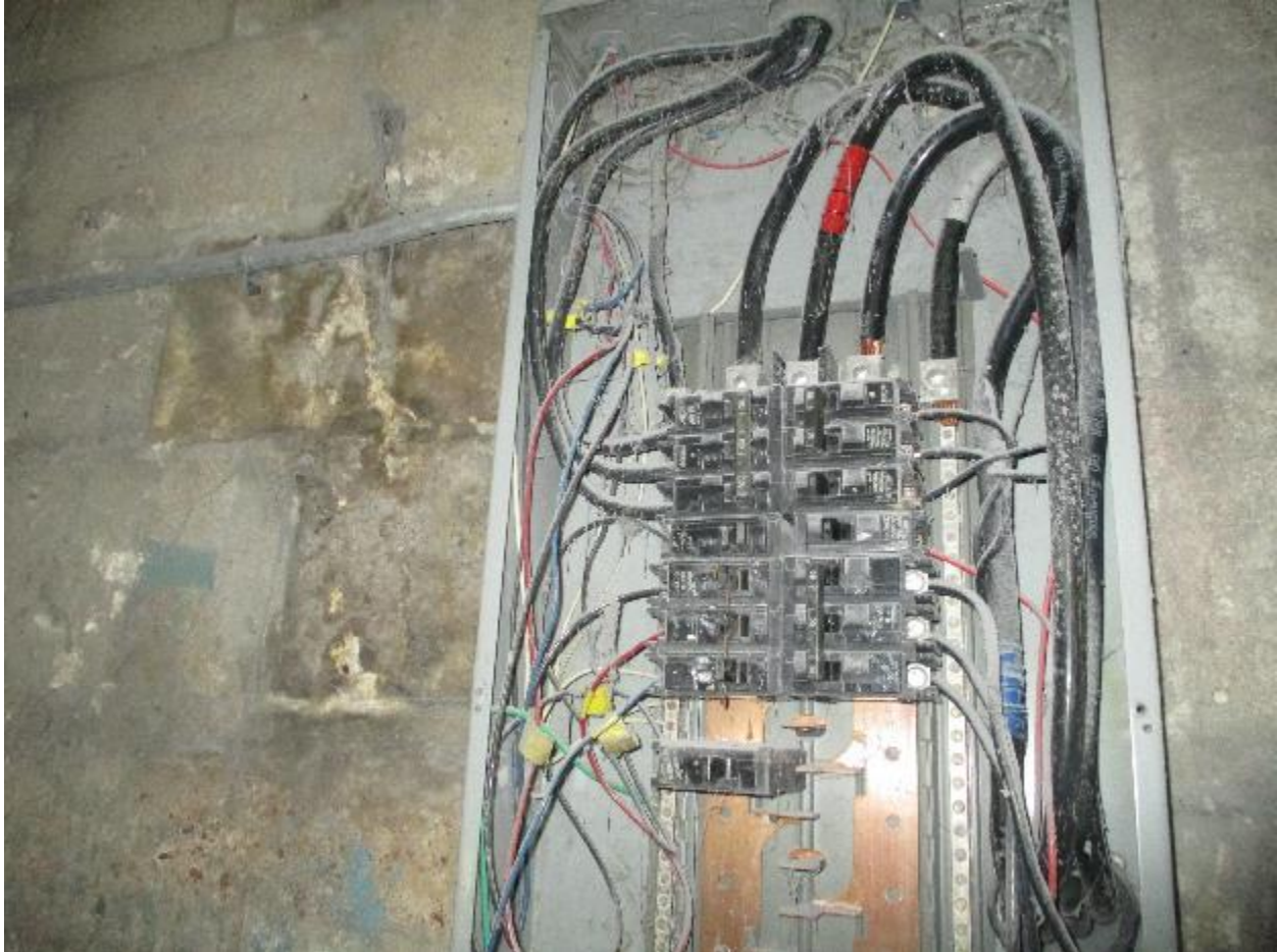
Electrical breaker panel in good condition at the time of inspection.
