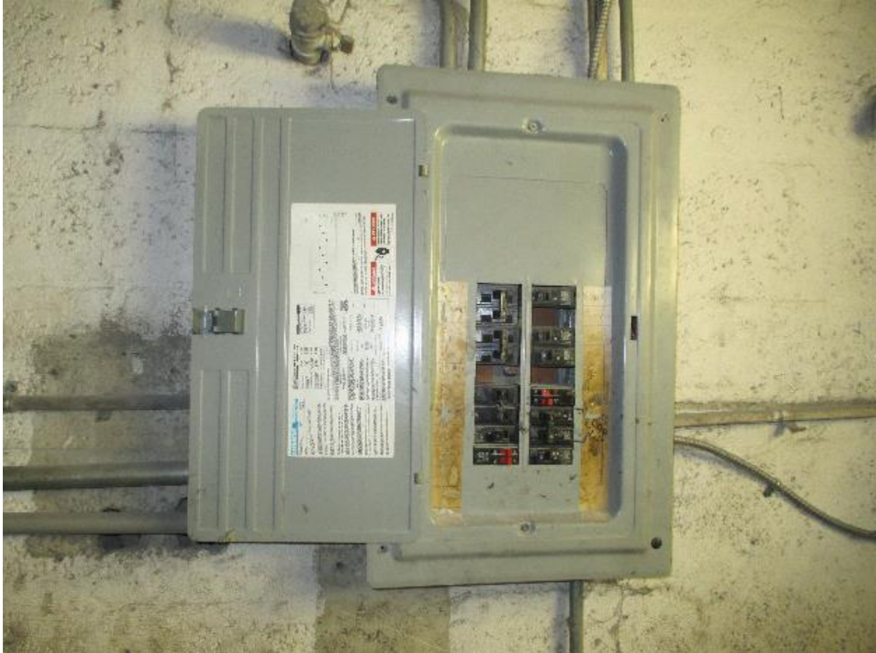
Electrical wires / Breaker panel double tap noted during inspection.
