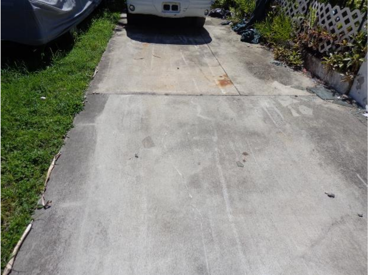
Driveway requires pressure wash.
