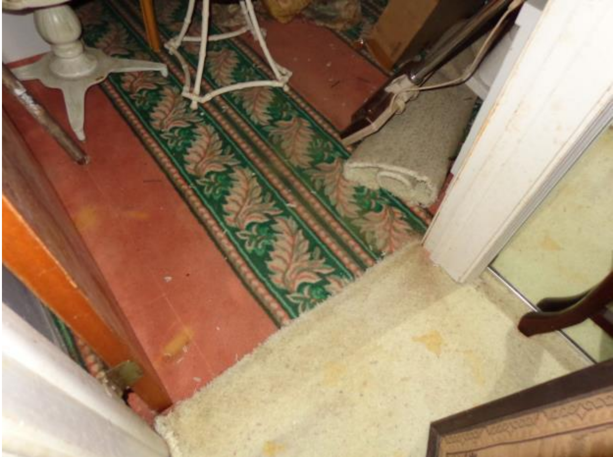
Soiled carpet throughout requires replacement.
