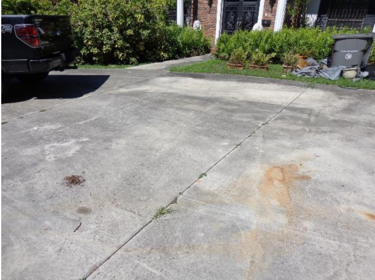
Driveway requires pressure wash.
