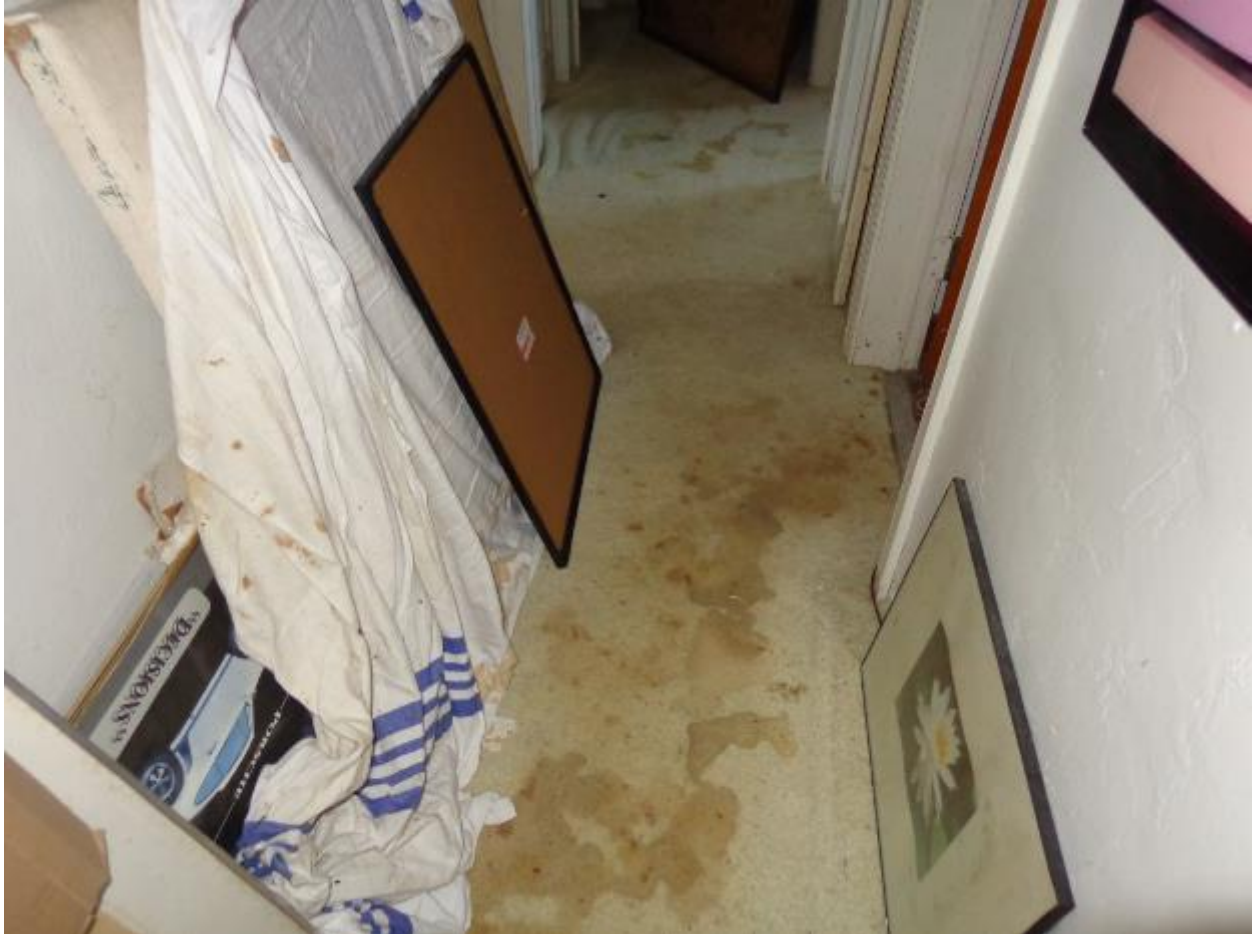
Soiled carpet throughout requires replacement.
