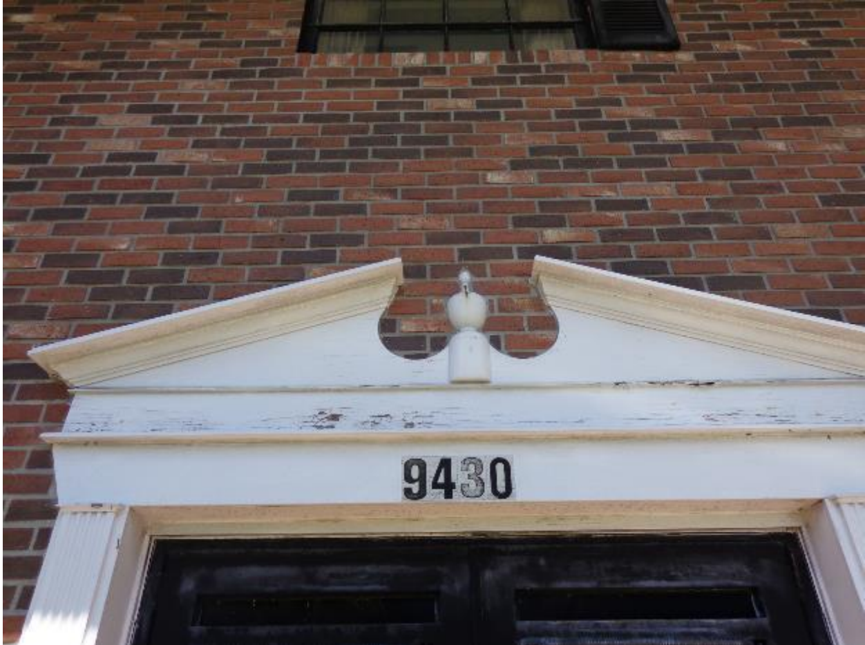
Rotted wood requires replacement.
