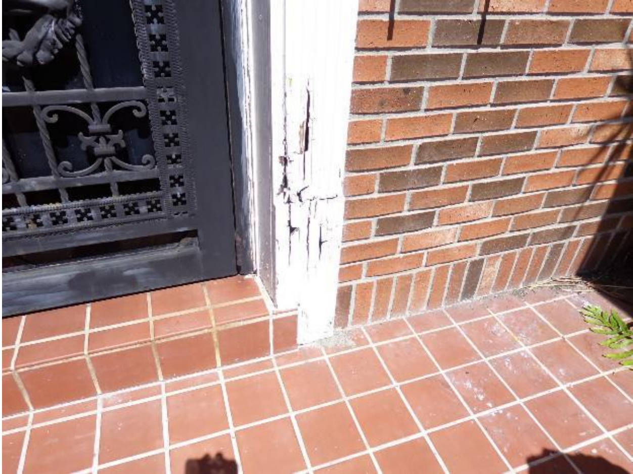
Rotted wood requires replacement.
