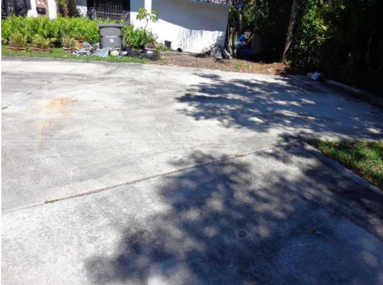
Driveway requires pressure wash.
