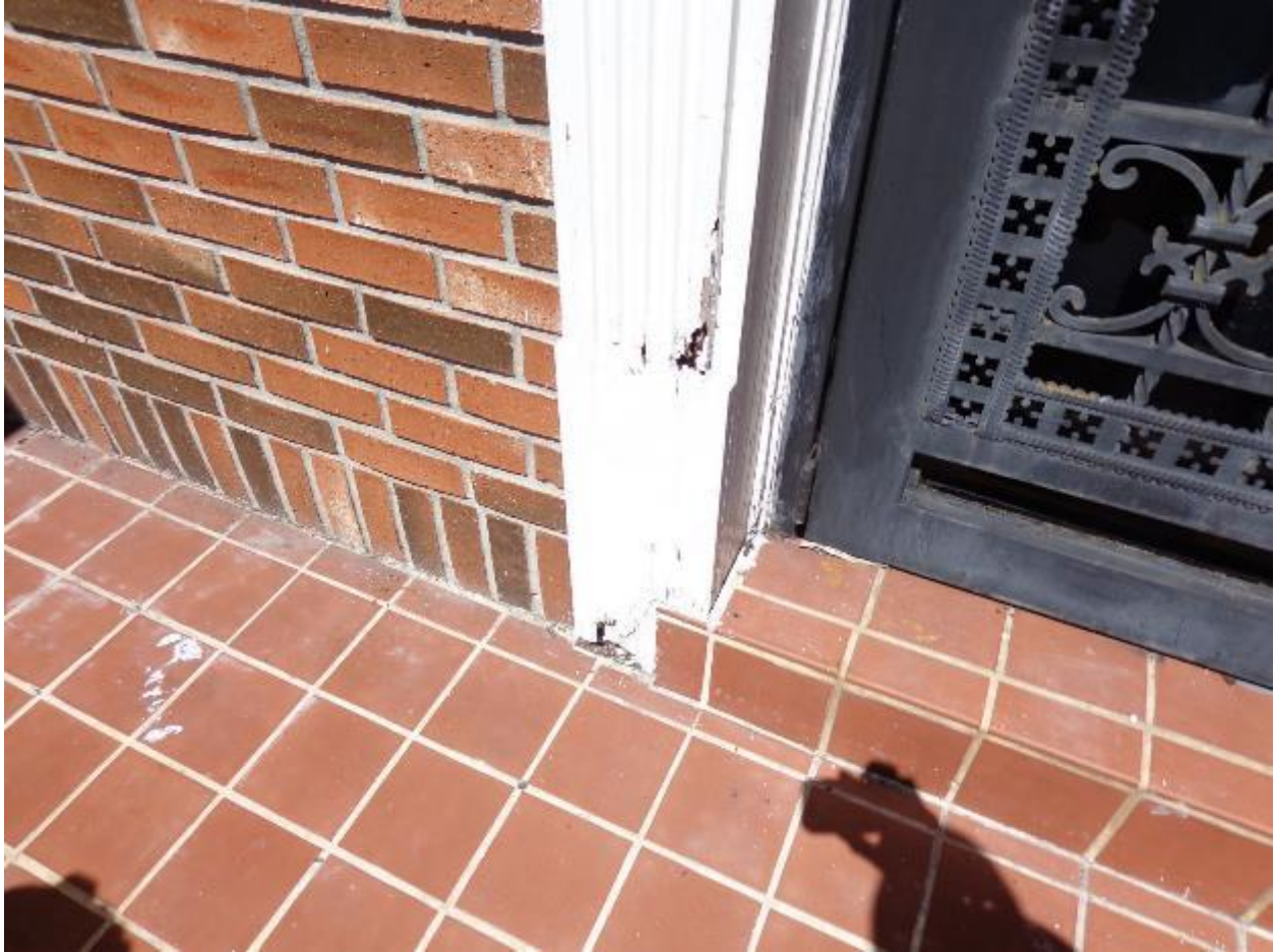
Rotted wood requires replacement.
