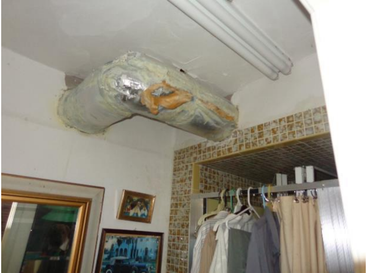
Duct work repairs required.
