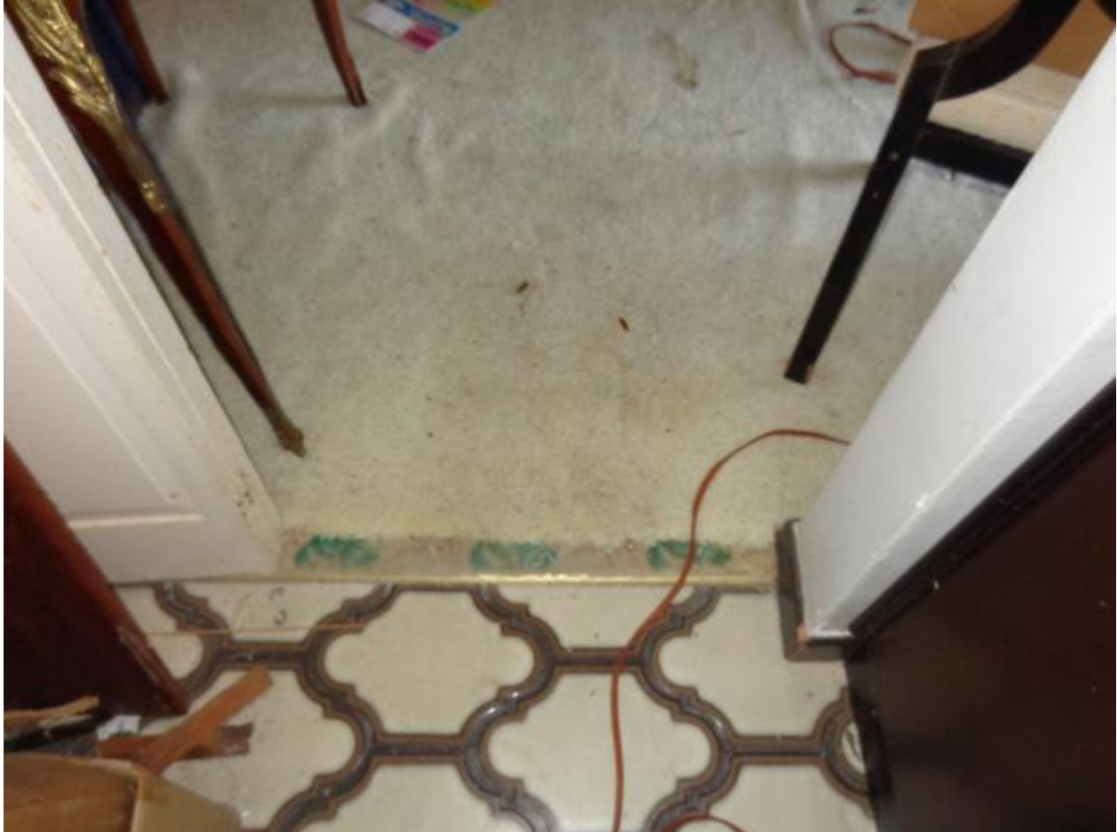
Soiled carpet throughout requires replacement.
