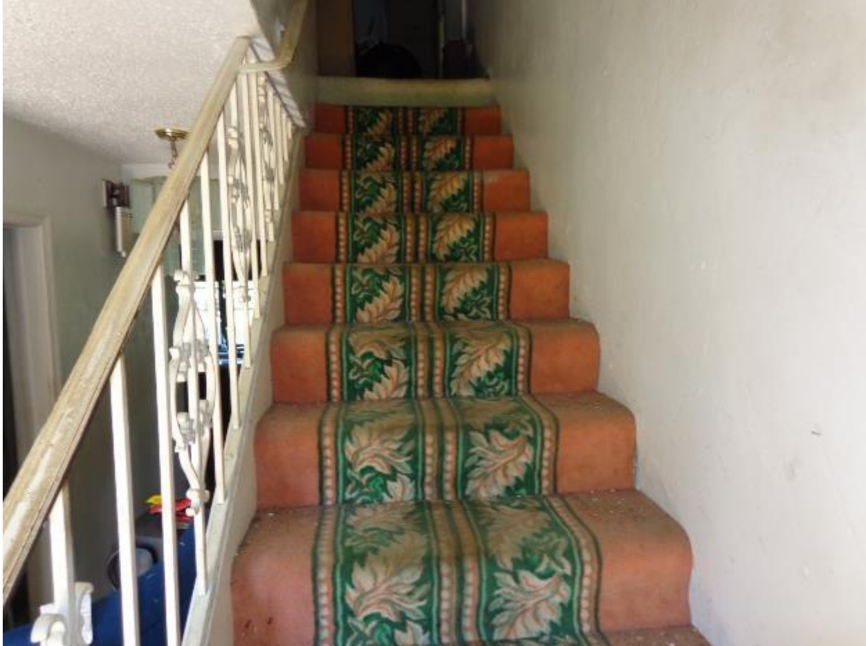
Soiled carpet throughout requires replacement.
