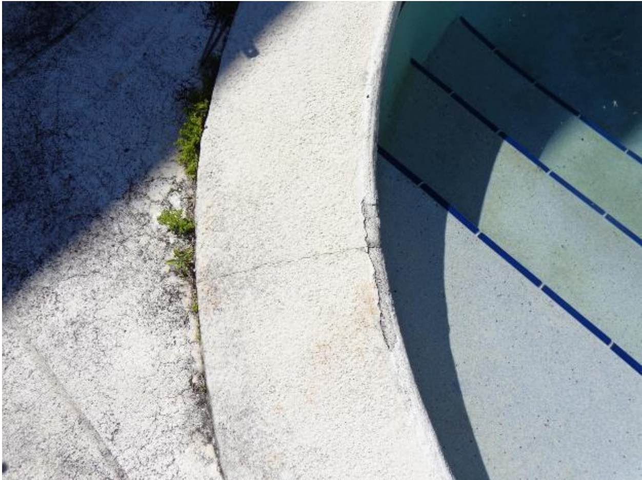
Pool deck requires structural repairs and resurfacing (concrete).
