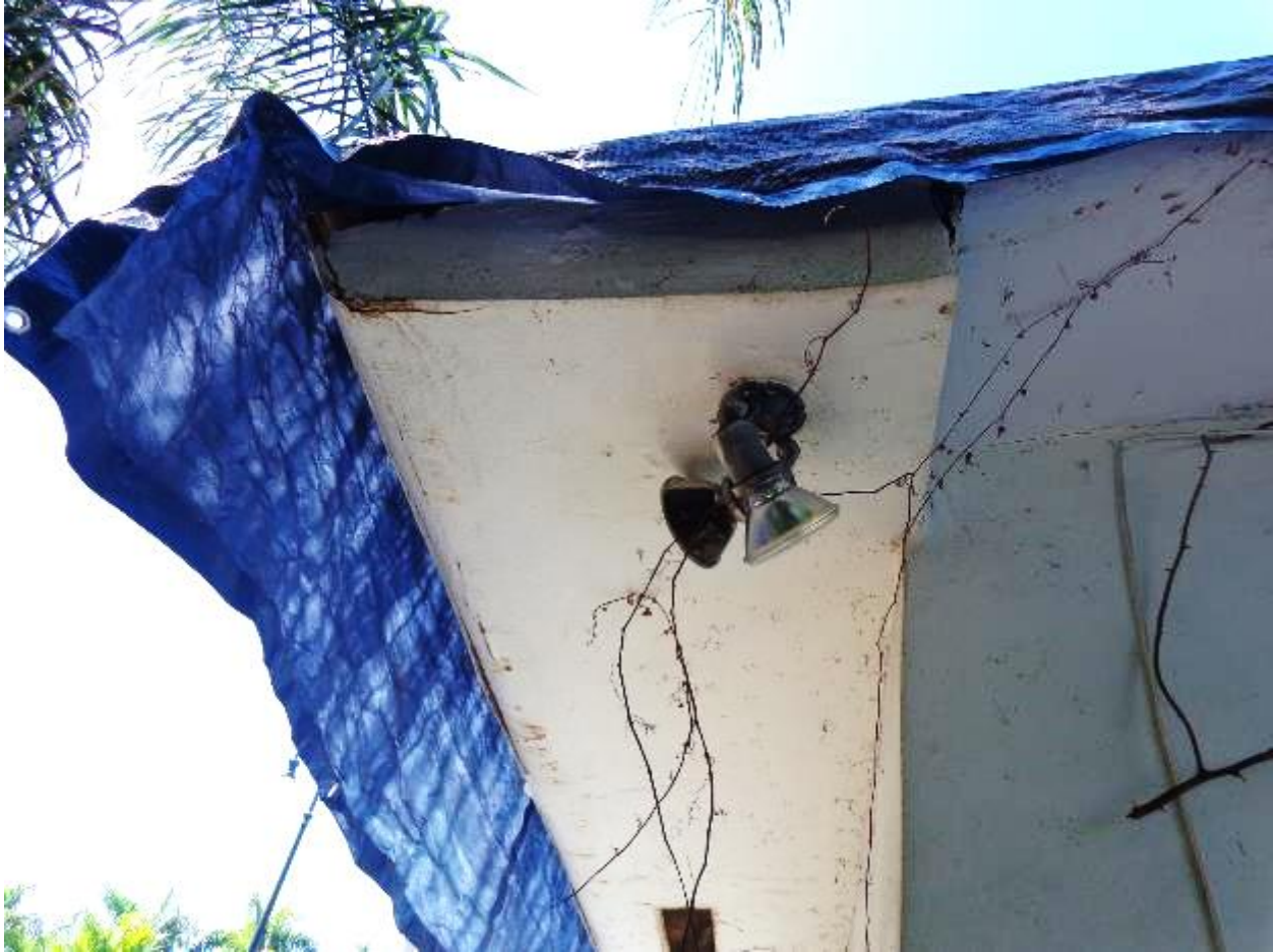
Stucco repairs required.
